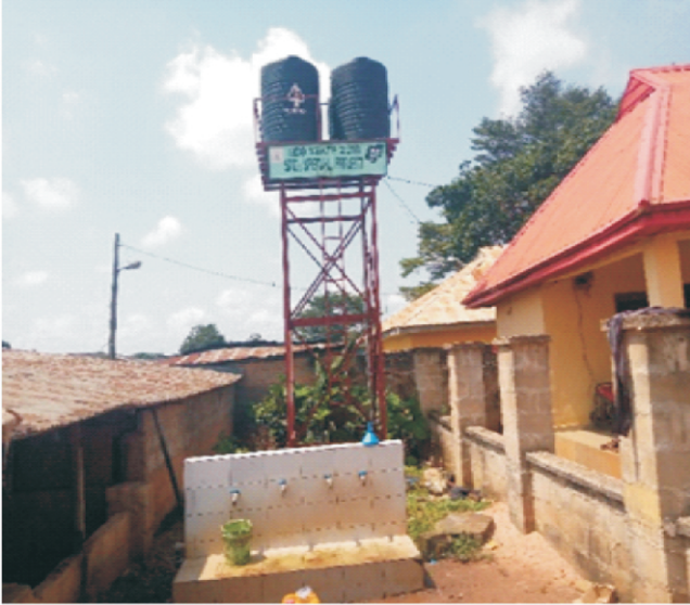
Plate 1: Water source at Uselu market
