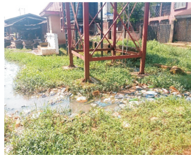
Plate 6: Poor sanitation at Ogida market
